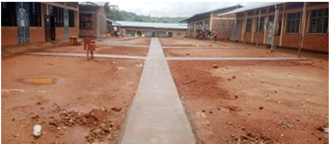
Improved walkways around the school site
